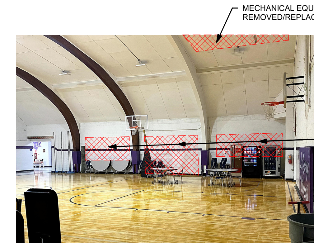
MECHANICAL EQUIPMENT TO BE REMOVED/REPLACED - SEE MECH CREATE NEW OPENINGS IN EXISTING MASONRY WALL. JAMBS OF NEW OPENINGS TO ALIGN WITH EXISTING FILLED IN WINDOW OPENINGS
